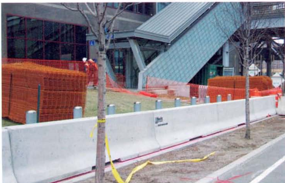
Barriers protect WTC transportation hub.
