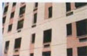
The architectural panels at the 32-story Marriott executive office building are buff-colored with a light acid wash and a precast brick accent feature.
