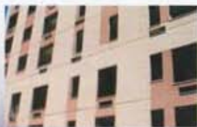
The architectural panels at the 32-story Marriott executive office building are buff-colored with a light acid wash and a precast brick accent feature.
